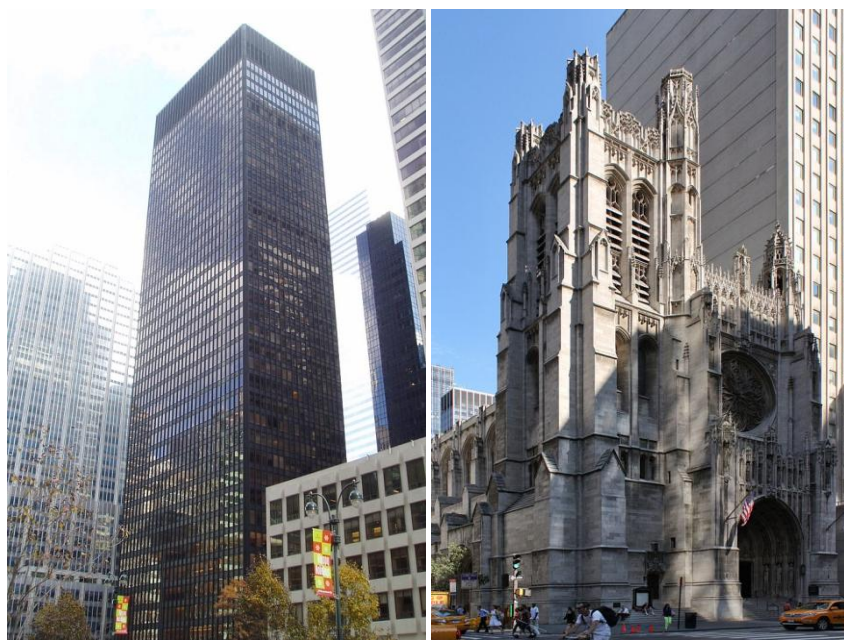
Fig.4_Da sinistra: Seagram Building, 375 Park Avenue, New York City e St. Thomas Church, 1 West 53 rd Street, New York City
