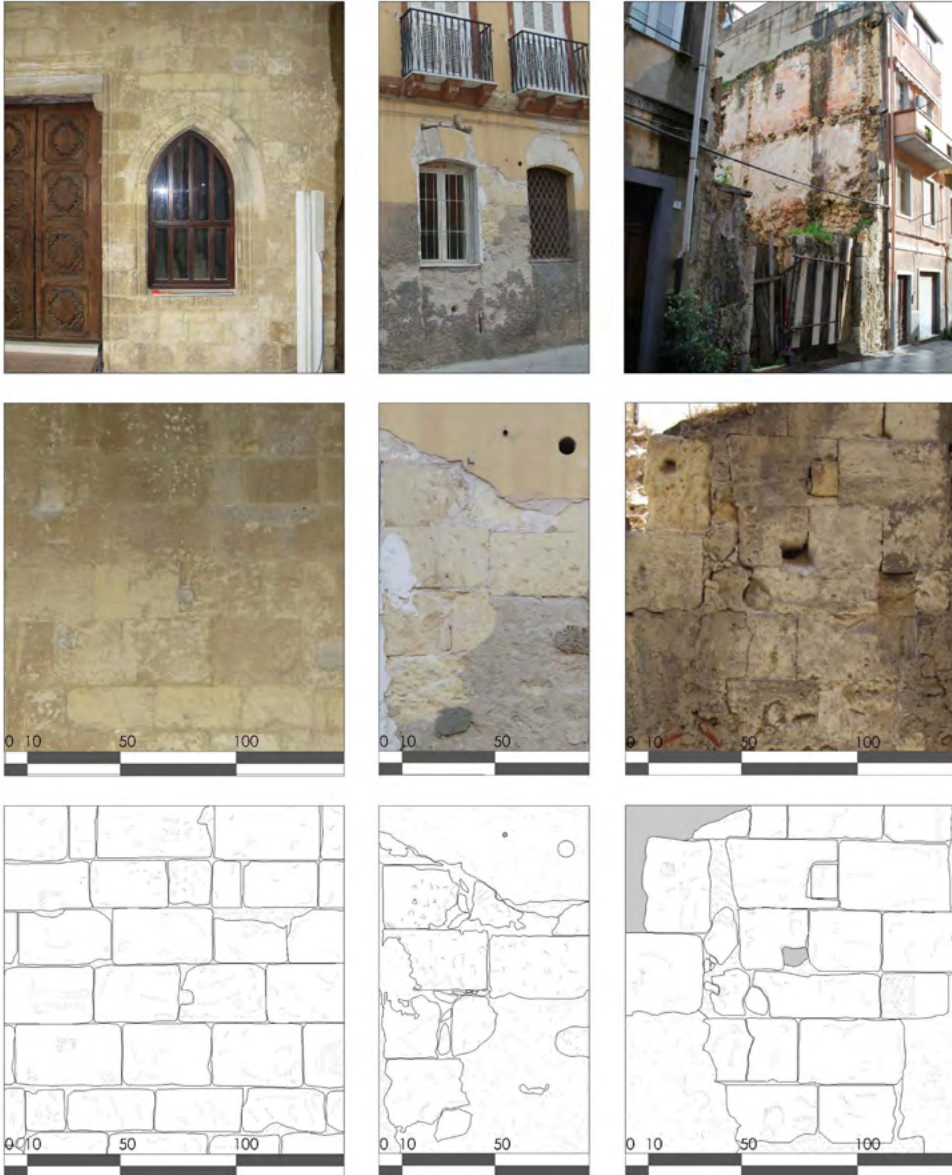
Figure 28. Other masonry-technique samples that show the same building technique M01, found in Santa Chiara. These can be found in other monumental and residential cases inside the historical centre of Cagliari (elaboration by E. Pilia).
