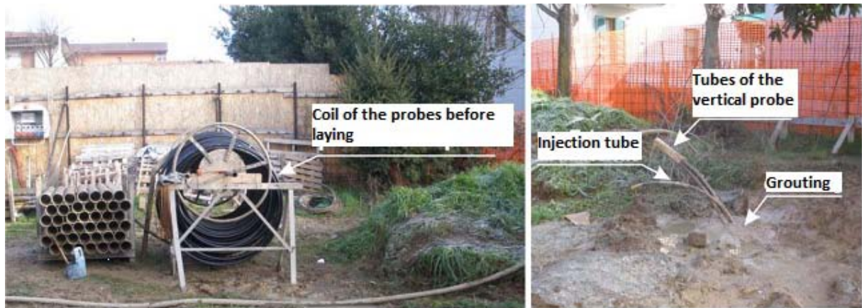
Figure 1.13 - Operations before the installation (left); probe after the injection of the cement (right).
