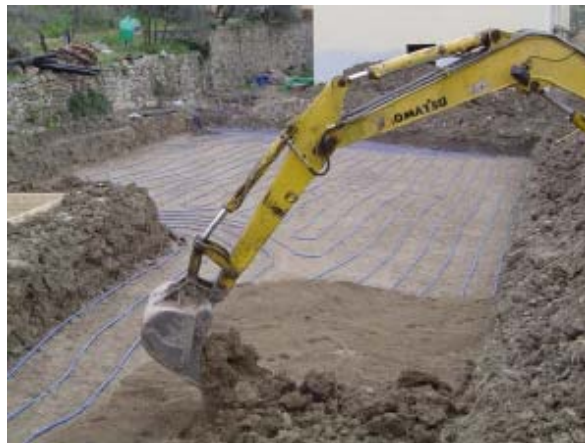
Figure 1.19 - Installation of the geothermal horizontal.
