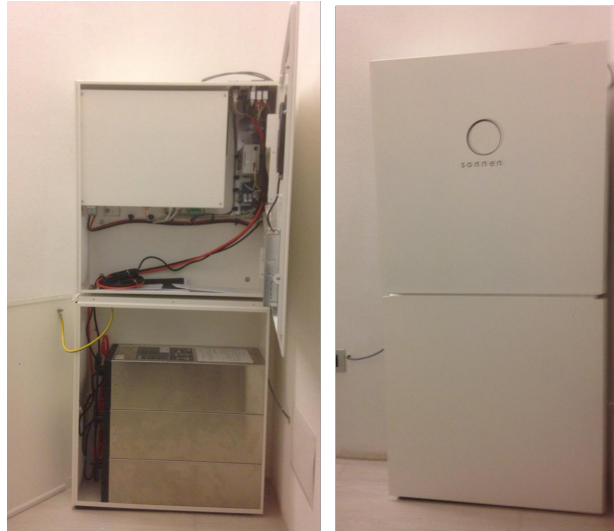
Figure 6.18: A energy storage systems that will be controlled by the VIRTUAL ENERGY VPP
