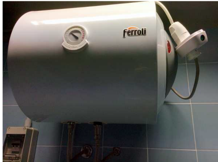
Figure 6.17: An electric water header connected to a smart socket integrated in the CoNetDomeSys testbed which will be part of VIRTUAL ENERGY VPP
