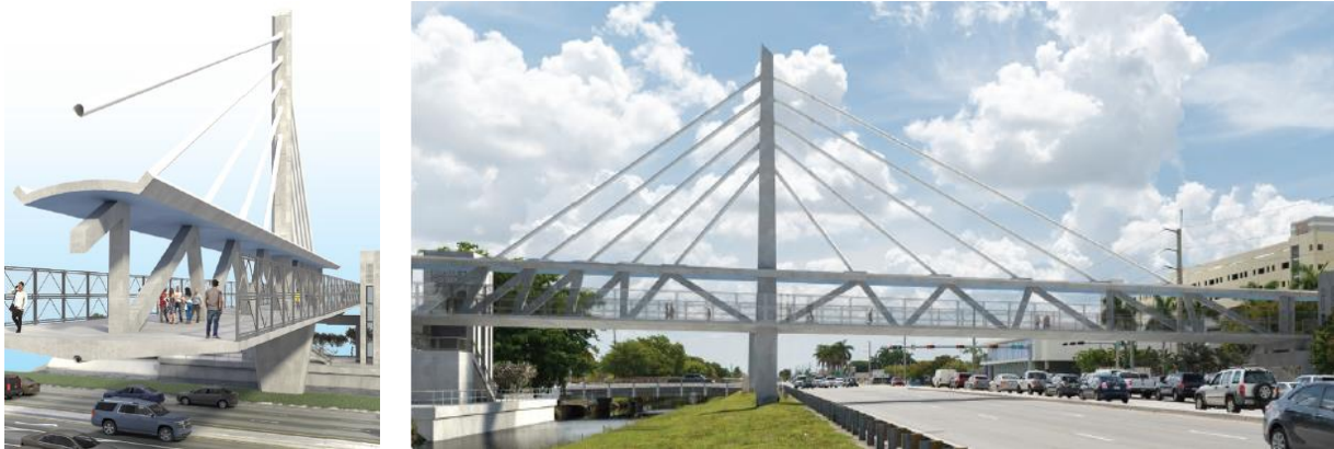
Figure 1: The analysed RC truss bridge [19].
