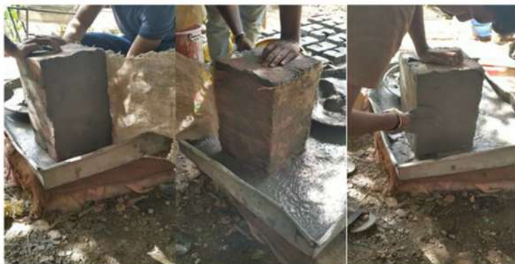
Figure 26. Jute fiber TRM retrofitting [96].
