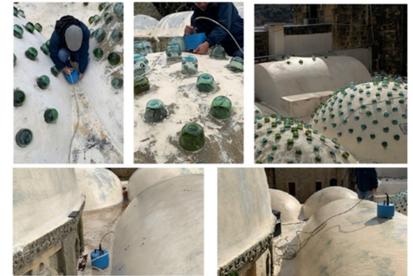
[Figure 148] Environmental modal tests and sensor installation on the roof.
