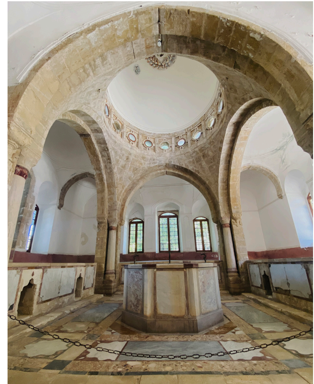
[Figure 141] Interior view of the main dome of B1, note the pointed arches, the dome with circular openings at the base and the common square base for the rectangular and L-shaped columns.
