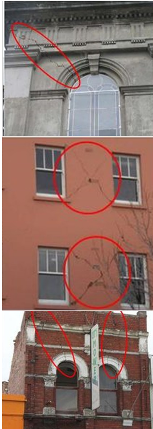
[Figure 7] Example of in-plane failure mechanisms (Dhakal, 2011).
