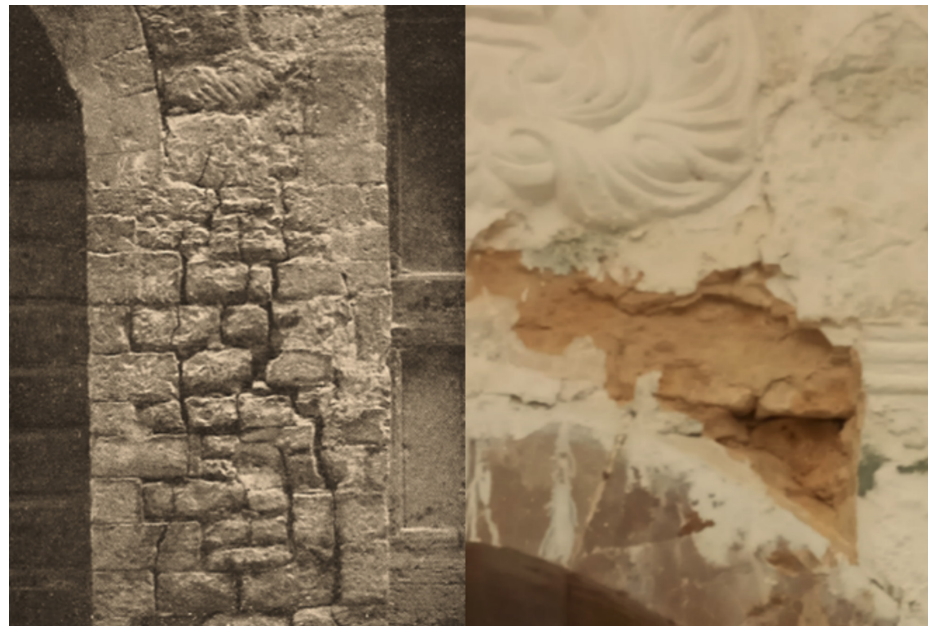
[Figure 5] Example of crushing of the material, photo to the right from (Angelillo et al., 2014).
