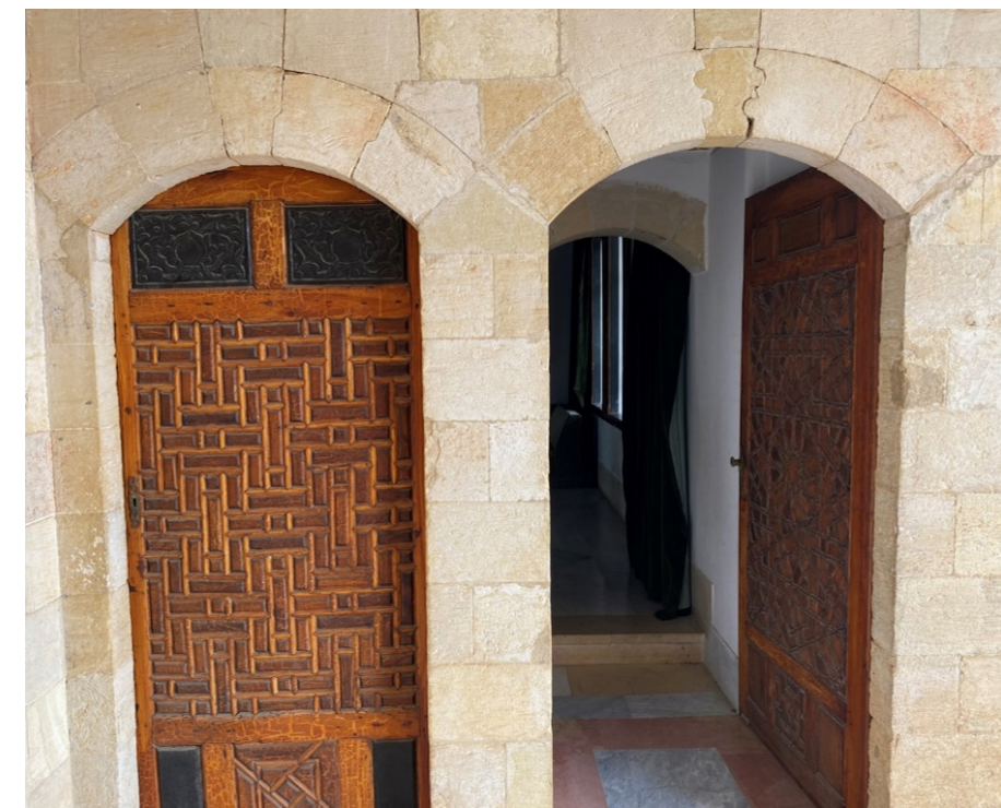
[Figure 43] Example of dual usage of the interlocking of voussoirs aimed for practical solution and decorative element in Beit El-Din, Lebanon a 19th century Ottoman masonry structure.
