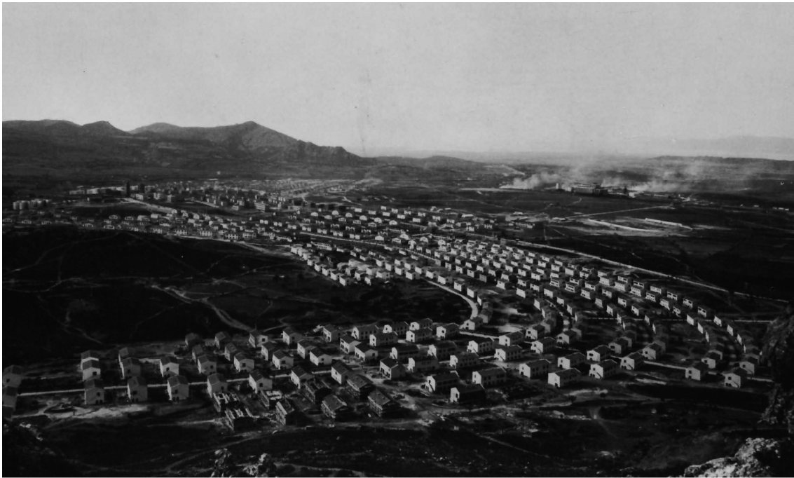
Fig.1 - Carbonia. View of the company town from the north, 1940
