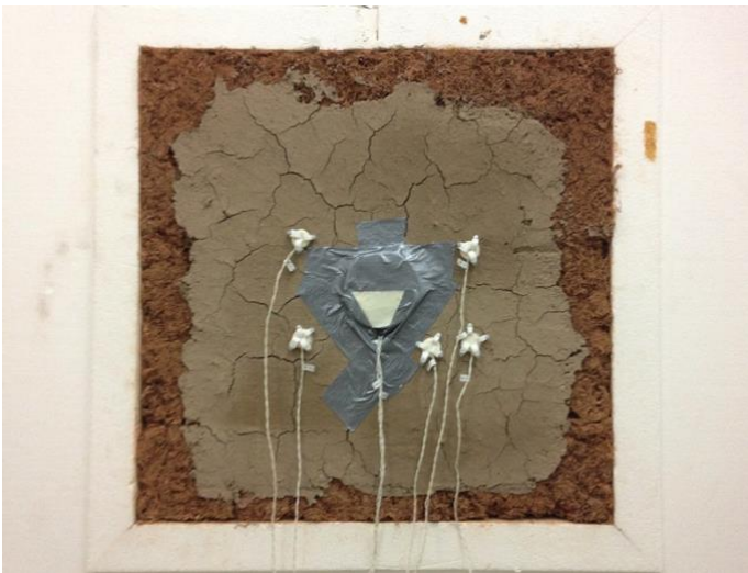
Figure 4. Straw-clay panels mounted on the ventilated roof
