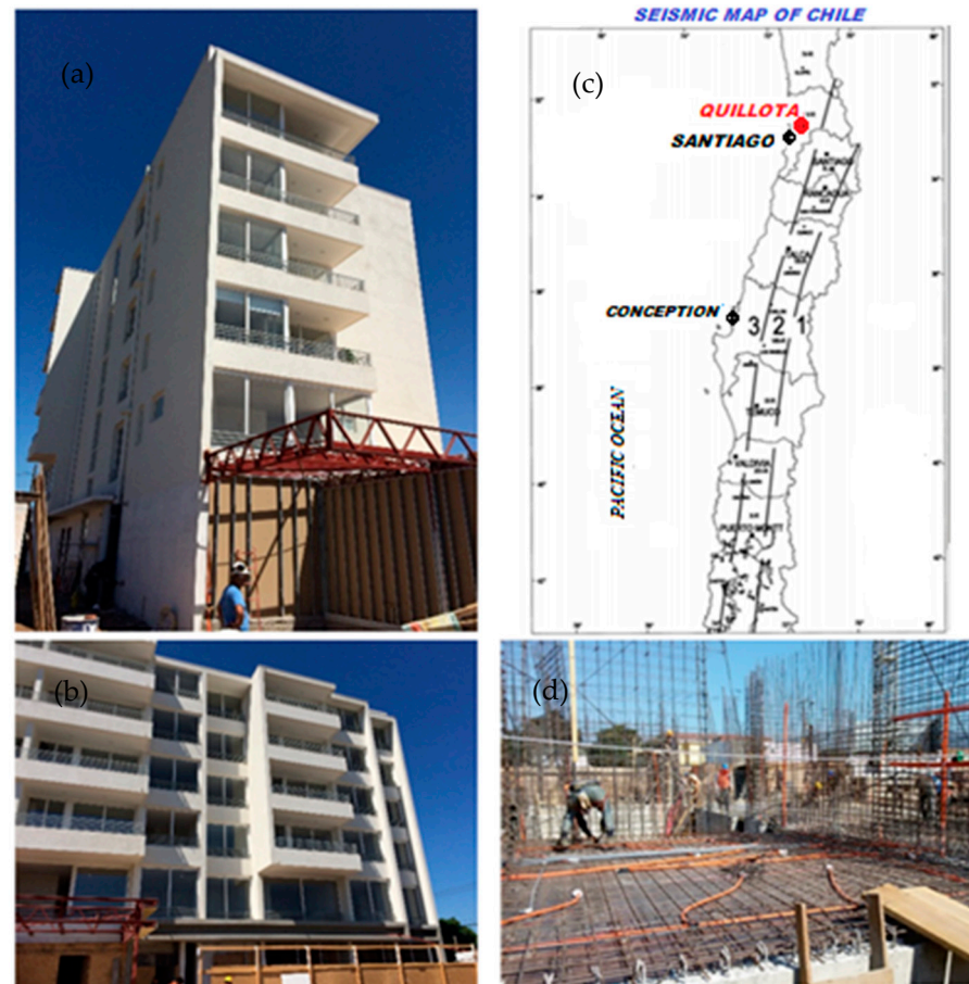
Figure 2. (a,b) Case-study building in the city of Quillota (c) seismic zones in central Chile. In the seismic map, Chile is divided into three bands numbered from 1 to 3, the latter being the higher seismic hazard band, to which Quillota belongs and (d) Details of the shear walls reinforcement.
