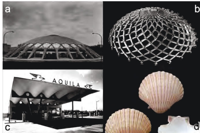
Figure 2: Example of corrugated shells: (a) Nervi's Palasport Flaminio dome, (b) Hobermann deployable structure, (c) Favini's roof, (d) corrugated sea-shells.
