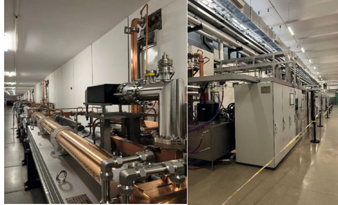
Figure 6.3.3.8: The HEPS linac tunnel and equipment corridor.
