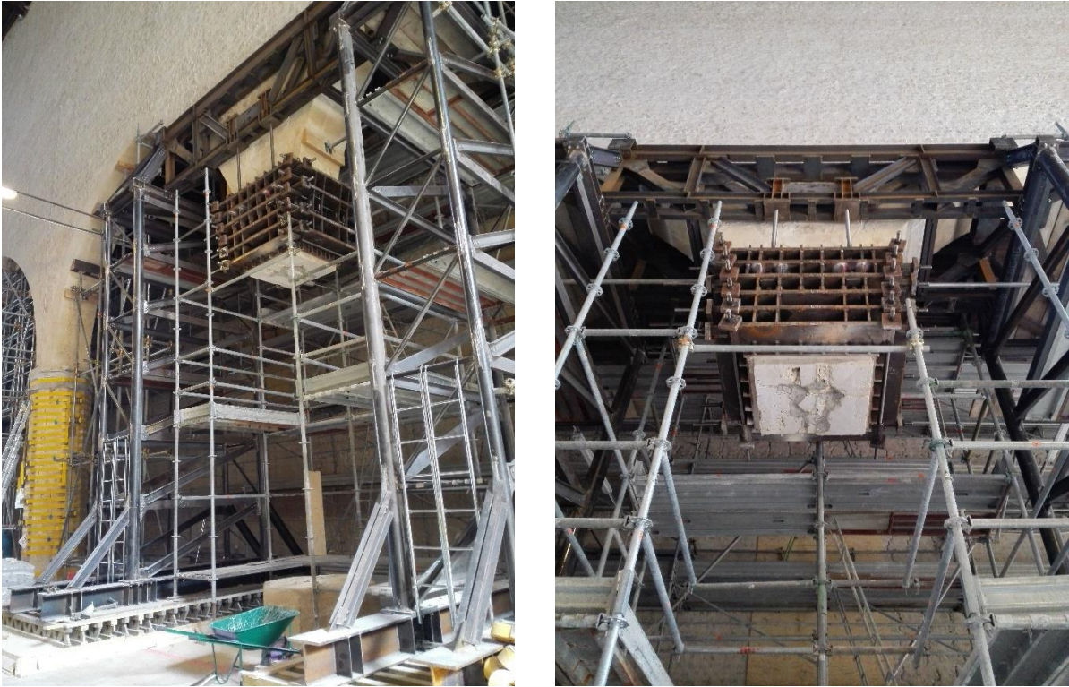
Fig. 13. The clamping system: disassembling of the column.
