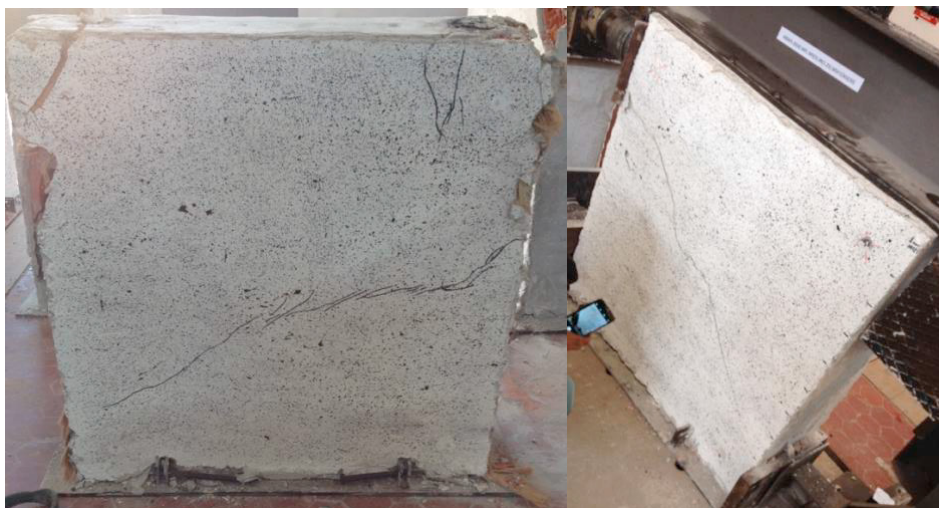
Fig 3. Typical failure pattern of strengthened wall showing diagonal crack.
