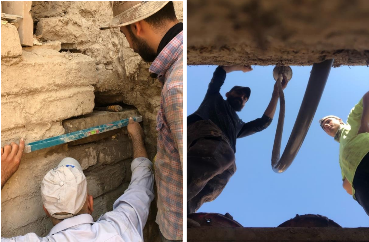
Photo 9. Wall stitching and earth grouting. Credits: M. Achenza
