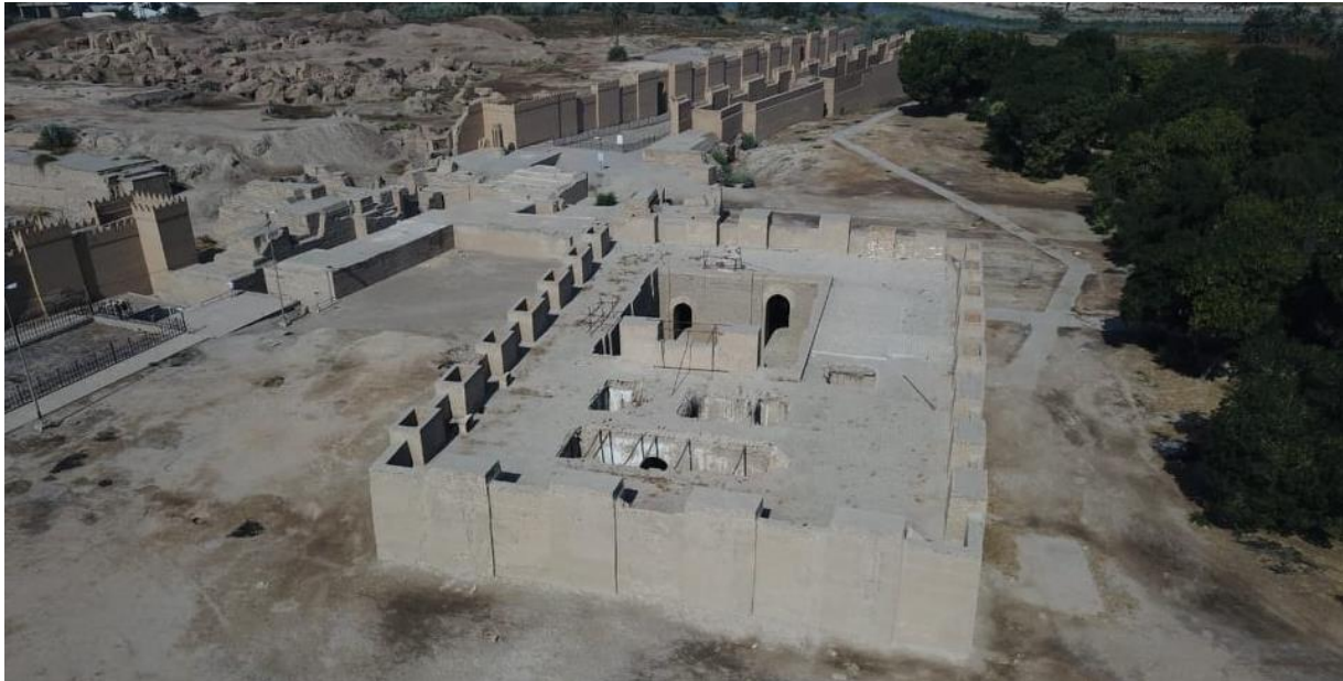
Photo 1. View of the temple of Ninmakh to the right of the Ishtar Gate and the processional way. Credit: Ammar Al Tae
