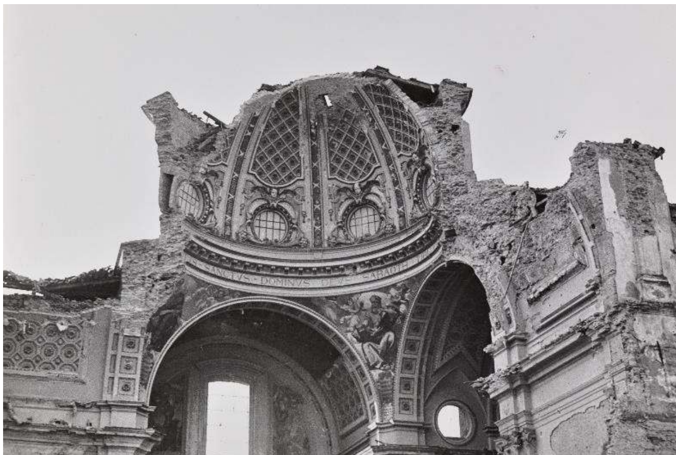
2: Detail of Dome of San Tommaso, Ortona, condition in spring 1944 after severe war damage [College Park, NARA, RG 239-PA, no copyright restrictions].
