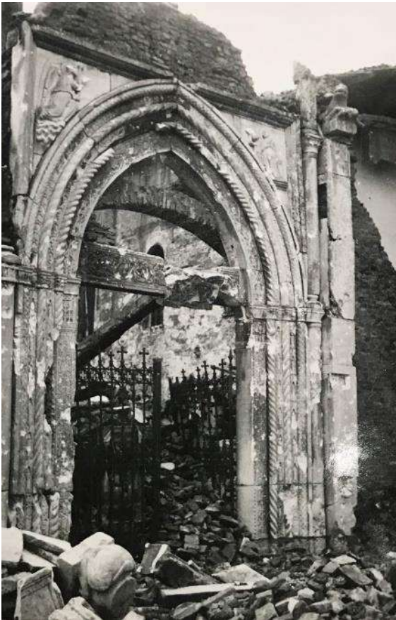
1: Gateway of San Giovanni Evangelista, Ravenna, first half of 14 th century; condition in Dec. 1944 after war damage [College Park, NARA, RG 239-PA, no copyright restrictions].
