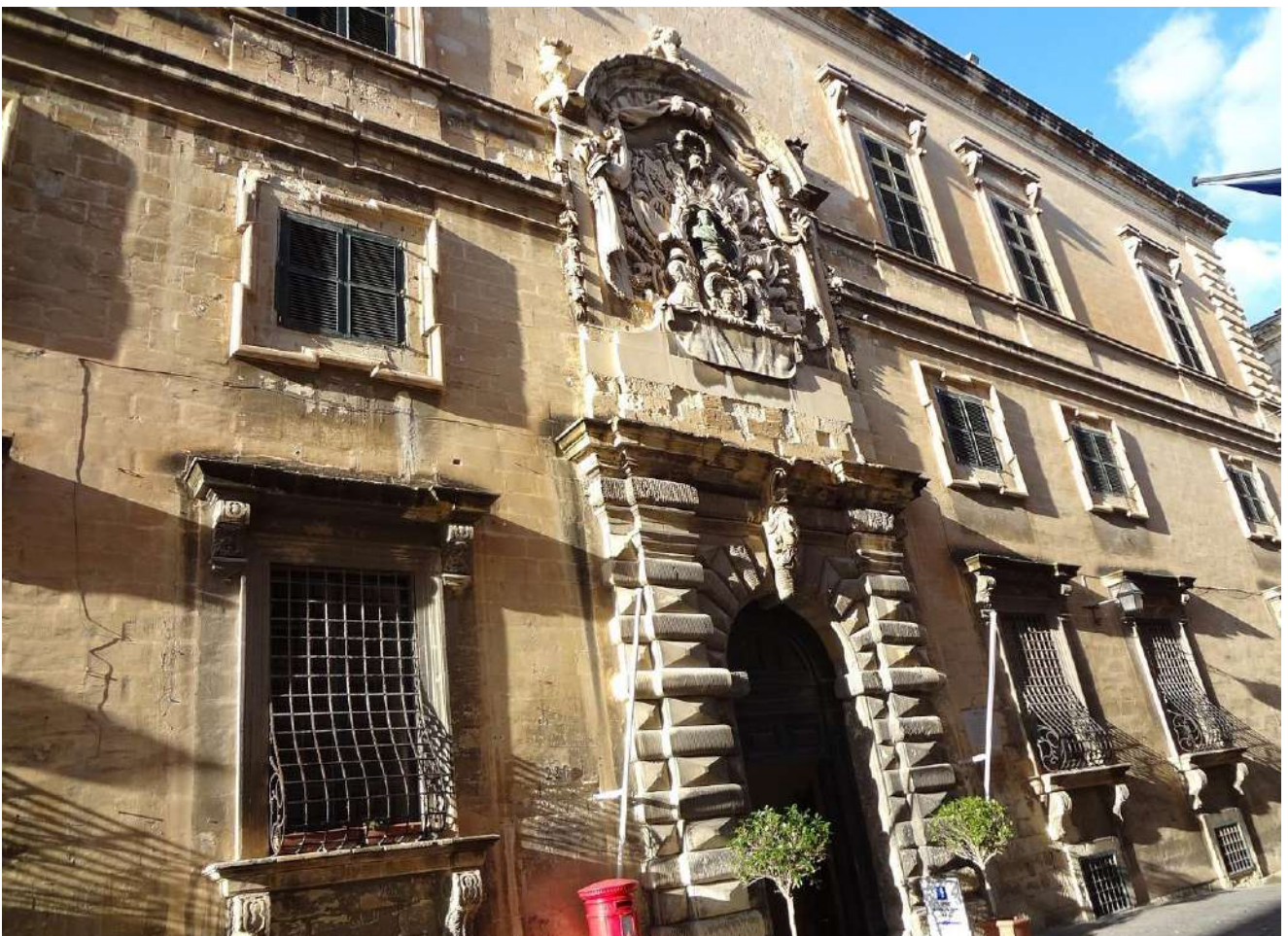
3: Façade of the Auberge of Italy [V. Burgassi 2022].
