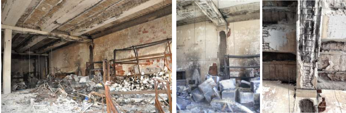
(a) (b) (c) Figure 5. Damages inside the warehouse: (a) overview, (b) column, (c) beam.
