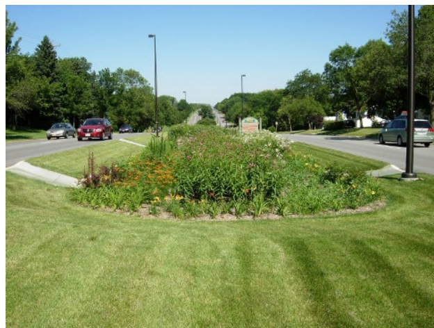
Figure 3: Retention basin of Grange Avenue in Greendale, Wisconsin. Source: Aaron Volkening, [CC BY 2.0]. Retrieved from Sgobbo, 2018.
