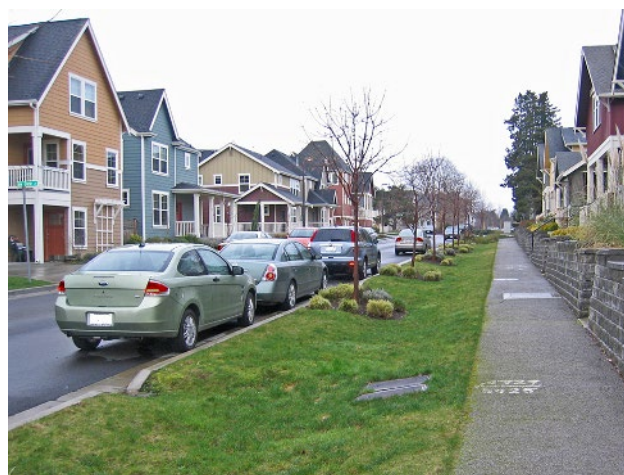
Figure 4: Runoff garden in High Point, Seattle, Washington 2010. Source: Brett VA, [CC BY 2.0]. Retrieved from Wikimedia Commons.
