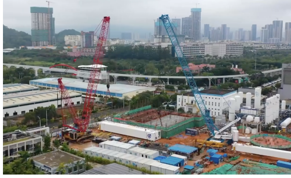
Figure 6: Cooperative hoisting with two crawler crane produced by Sany.
