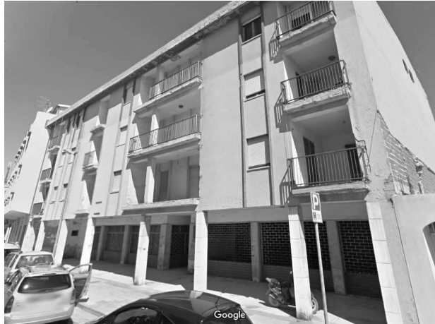
Fig. 6: Front view of the council housing building
