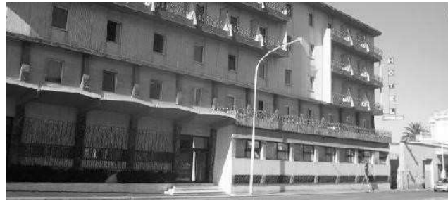
Fig. 2: Front view of the hotel
