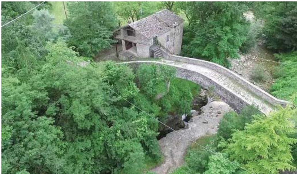
Figure 1: Aerial view of the bridge
