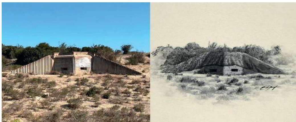
Bunker near Lake Simbirizzi: photograph and reconstruction drawing of the camouflage arrangement (1942–43). Graphic elaboration: Giancarlo Sanna.
