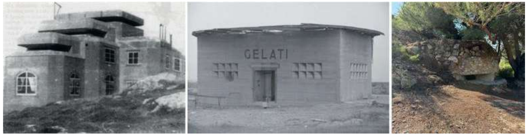
Fig. 2. Anthropic camouflage on military architecture. Comparison of cases in France (Atlantic Wall), Italy (Rimini), and Spain (Clot de Galvany): simulations of ordinary architectures and “identity-shift” strategies (collage). Image sources: Fig. 2a–c.
