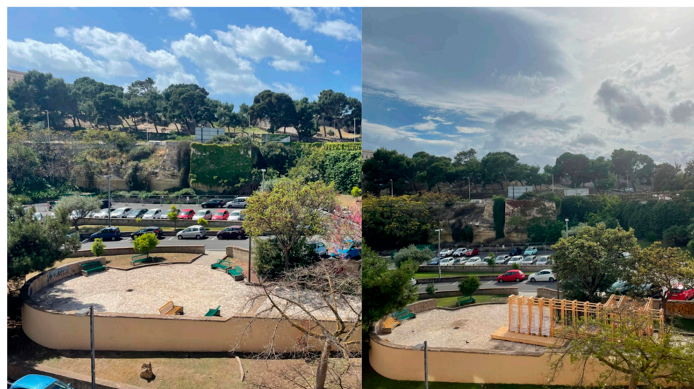
Figure 2. Site A is shown in two images: on the left, the site before the self-construction intervention, and on the right, the same site after the intervention.
