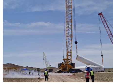
Fig. 2. Cooperative hoisting of wind turbines with two crawler cranes.
