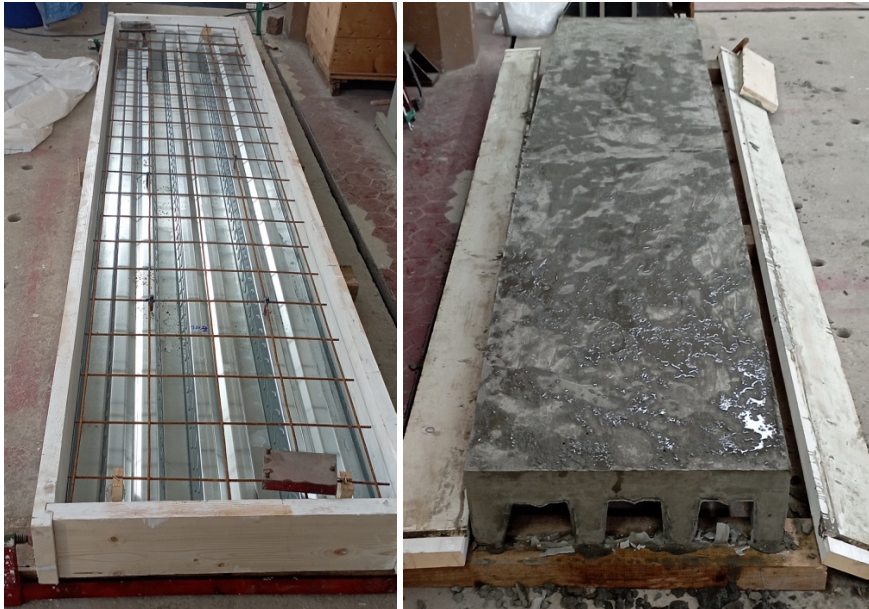
Figure 1- Composite slabs before (left) and after concrete casting (right).
