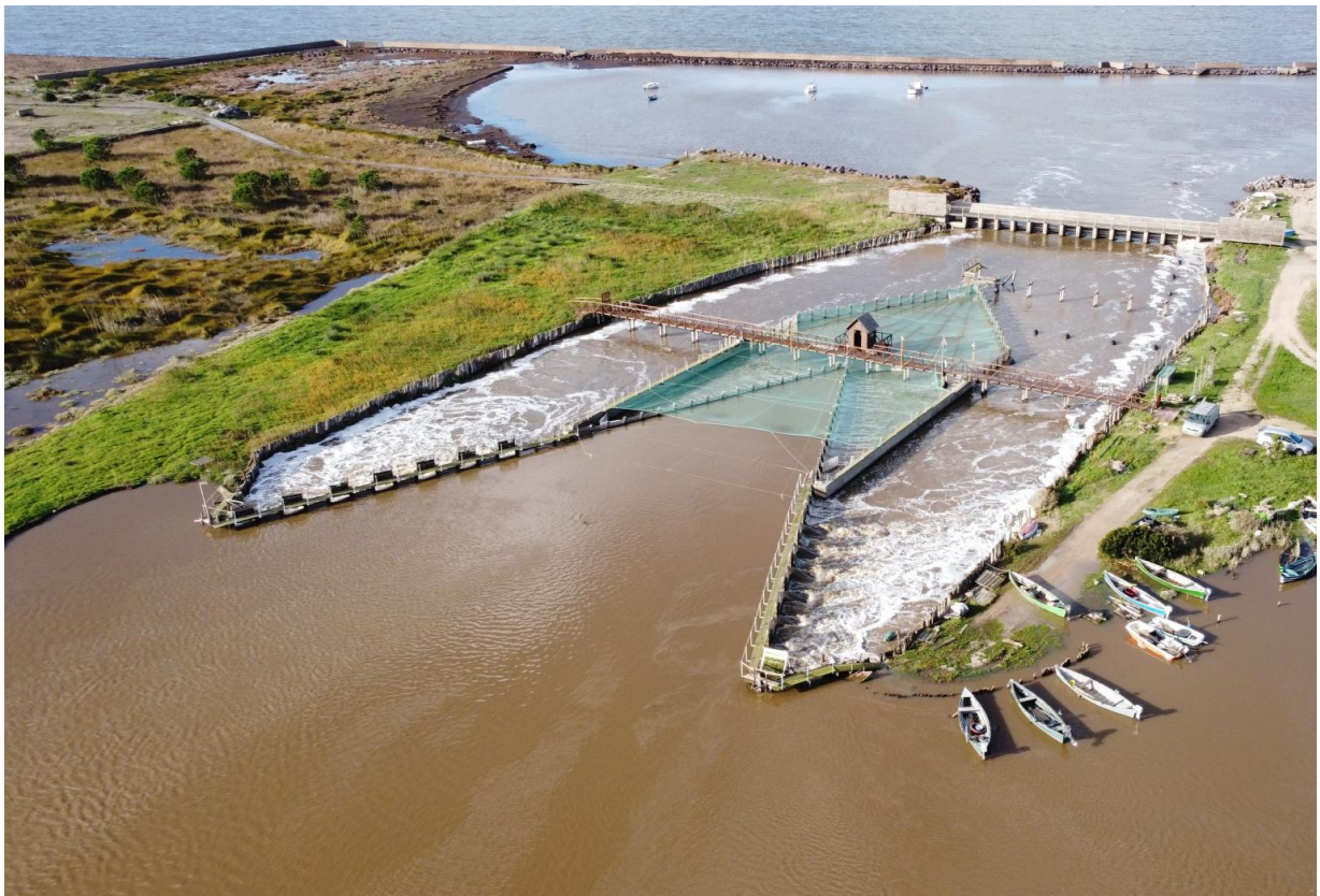
Figure 4.4 Flooding event in S'Ena Arrubia lagoon in 2020 (Photo provided by Cooperativa Sant'Andrea; Ph. Alessandro Porcu).
