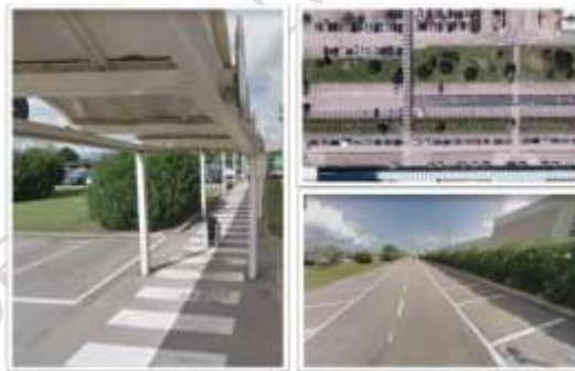
Fig. 11: Covered shelters connecting the long-term and short-term parking and Sector C - short-term parking and Loading/Unloading Stalls
