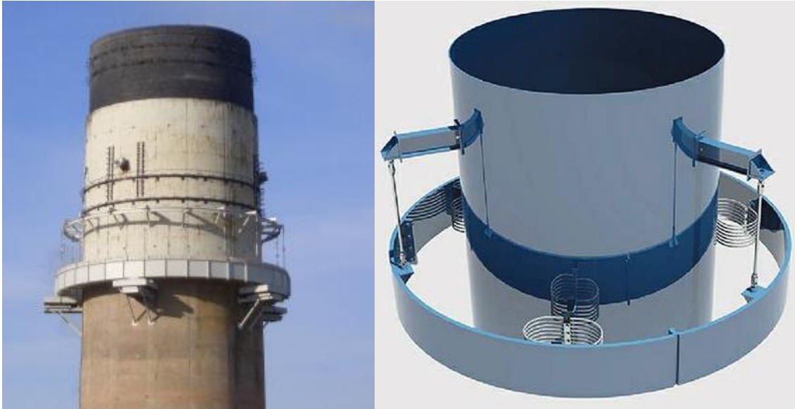
Fig. 1. World record for a 41 t tuned mass damper installed on the top of a 180 m RC chimney [48].
