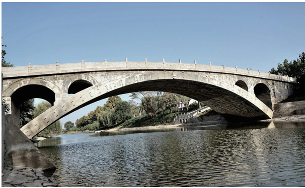
Fig. 3 Chinese arch bridges: Zhaozhou Bridge, Hebei province, China.
