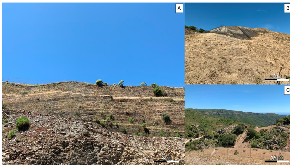
Figure 6. Remediation actions conducted at the Bacchu Locci mine. A) An overview of the tailings disposal facility, highlighting stabilization structures with mesh systems and implemented revegetation interventions; B) A detail of the interventions; C) Panoramic view of the mining area.
