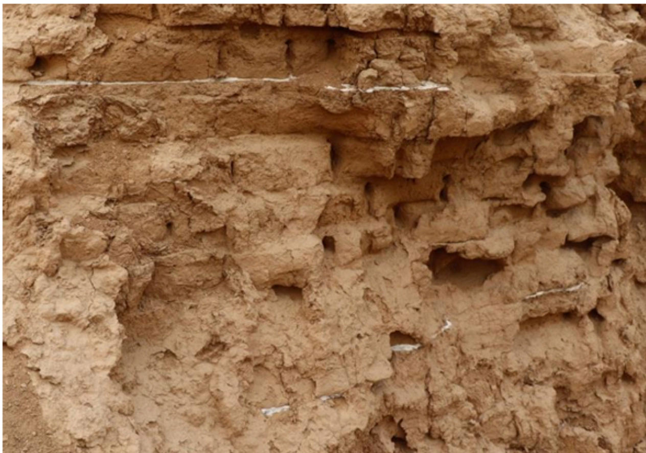
Figure 10. Borsippa: reed mats in earth masonry. Credits: Ammar Al Taeer
