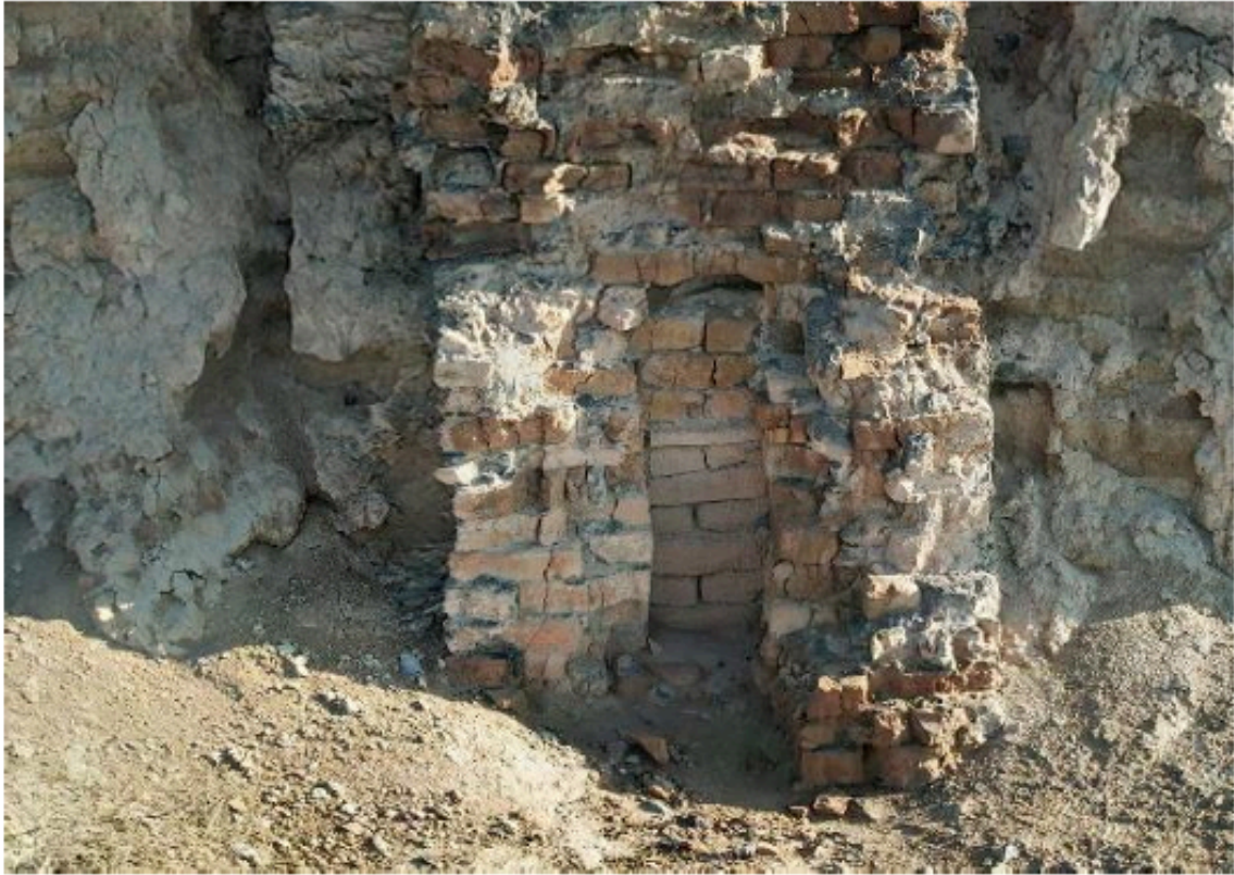
Figure 4. Water drainage in the Ezida Temple. Credits: Ammar Al Taei
