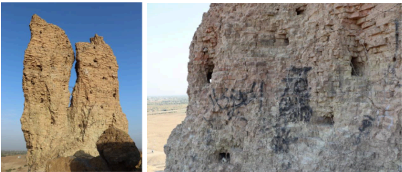
Figure 11. Ventilation channels in brick masonry. Credits: Ammar Al Tae
