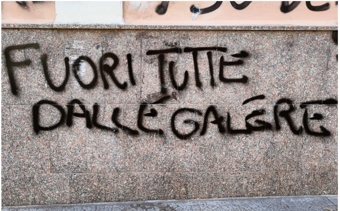
Figure 1. Example of graffiti vandalism on external cladding with Ghiandone granite in Sardinia (photo courtesy of S. Cuccuru).
