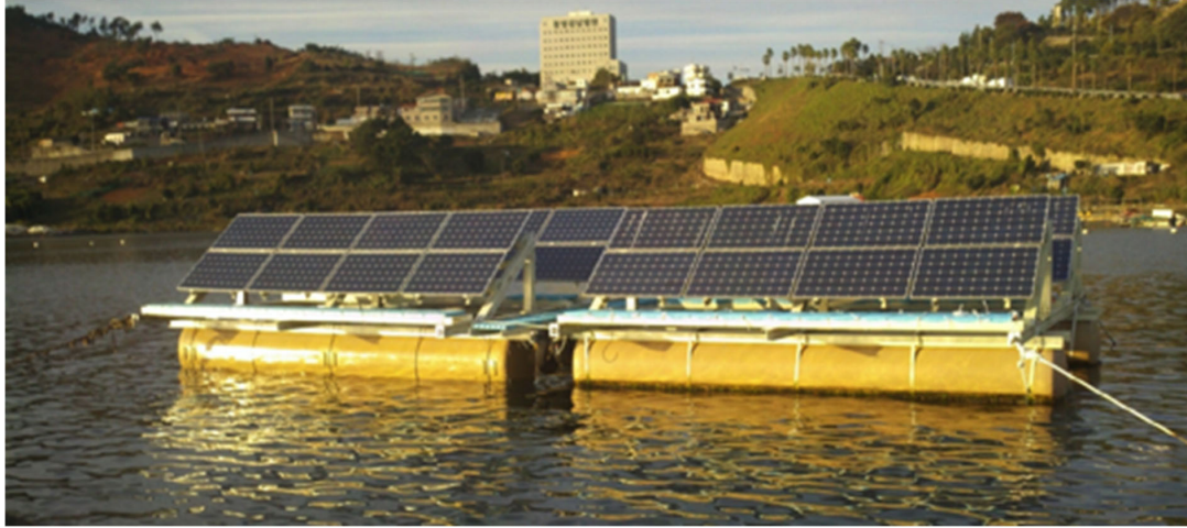
Figure 25. PV panels mounted on fiber-reinforced polymeric plastic structures placed on a floating system [81].
