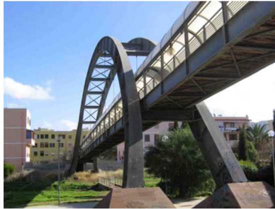
Fig. 6. The footbridge on Cannas River
