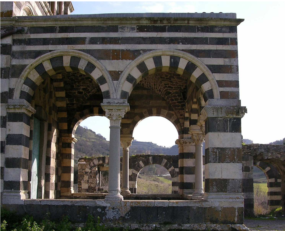
Fig. 4 – Trinità di Saccargia abbey. The western portico, with late 19th century granite columns which replaced the original limestone ones.
