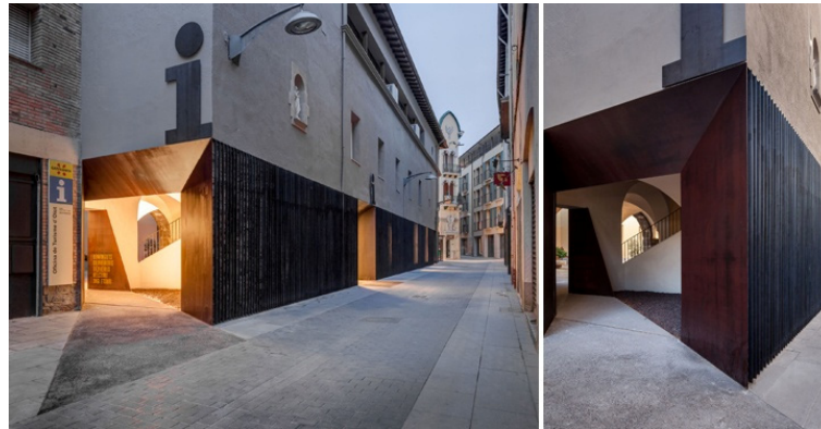
Fig. 2 Former Olot Hospital (Spain): ground floor accessibility.
