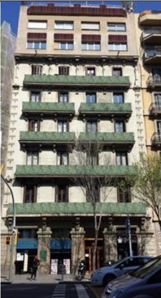
(C) Coloured polycrystalline glasses in the façade and in balconies
