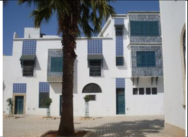
(B) Monocrystalline panels + coloured polycrystalline glasses in balconies
