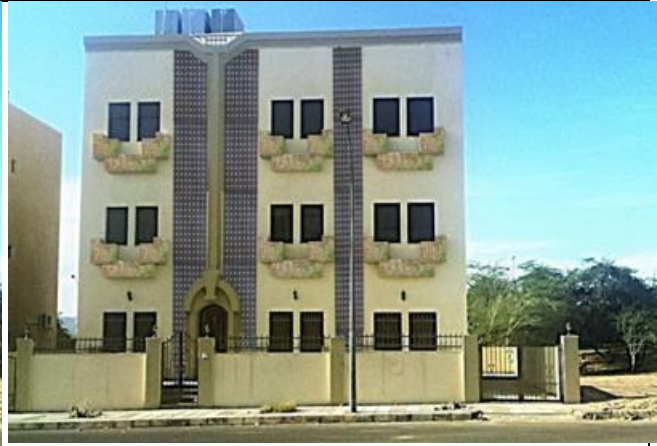
(B) Monocrystalline panels + coloured polycrystalline glasses in balconies
