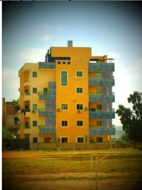
(D) Coloured polycrystalline glasses in balconies and a solar shading PV technology
