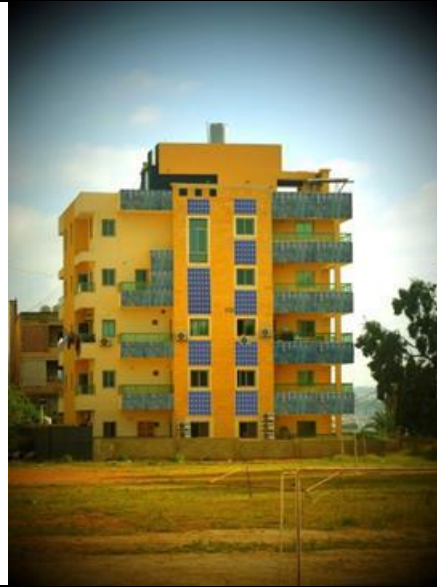
(B) Monocrystalline panels + coloured polycrystalline glasses in balconies
