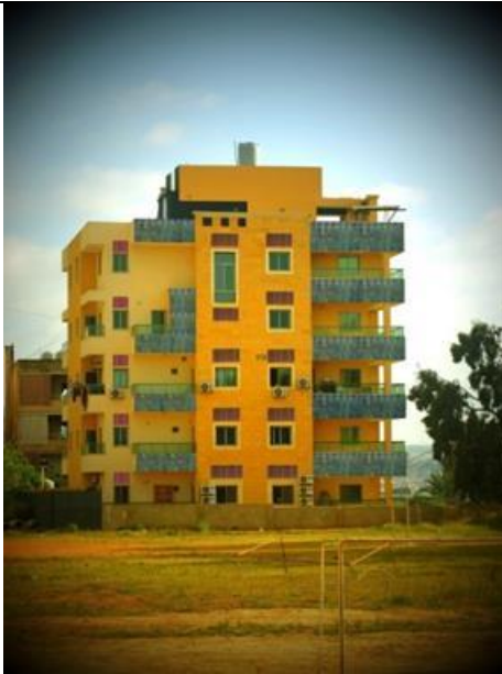
(C) Coloured polycrystalline glasses in the façade and in balconies
