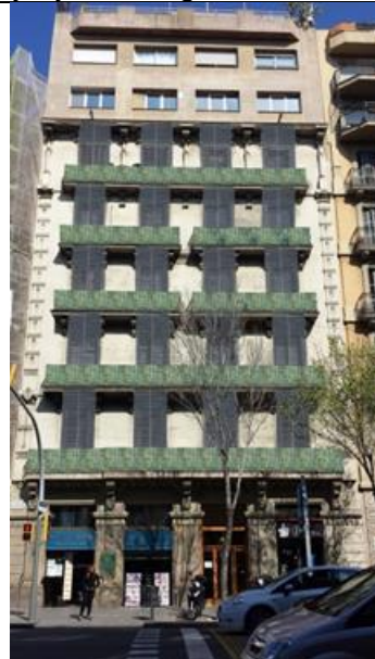
(D) Coloured polycrystalline glasses in balconies and a solar shading PV technology
