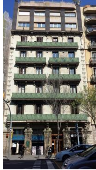
(B) Monocrystalline panels + coloured polycrystalline glasses in balconies
