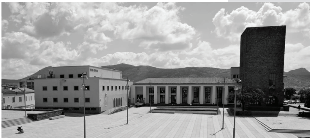
Figure 1. The OND building after restoration in late 2001 (picture of A. Sanna).
