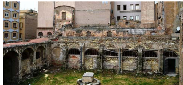
Figure 2: The buildings facing the cloister as seen from the north-east
