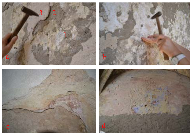
Figure 9: a) Sampling the different types of plaster found in the structure; three layers of plaster are recognizable (1 white, innermost, on wall; 2 dark gray, intermediate; 3 light gray, outer); b) detail of the oldest plaster layer; c-d) consecutive layers of plaster, up to 1 cm thick, placed on older layers, often still carrying the original paint
