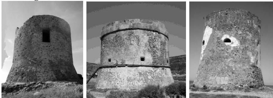
Figure 2. Argentina, Bosa and Pittinurri Towers. Photos: S.M Grillo
