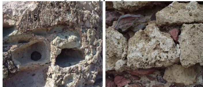
Figure 8. The Original Plasters of the Towers are Conserved in Some Places, as for Example in the Columbargia Tower (Right Side). When the Original Plaster is Weathered, the Mortar Very Quickly is Washed Out, Seriously Damaging the Stability of the Wall. On the Left Side an Example of Recent Restoration is Shown, Concerning the Argentina Tower. Photos: S.M Grillo
