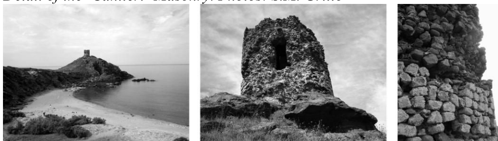
Figure 1. Columbargia Tower. Panoramic View of the Tower, its Structure and Detail of the ‘Cantieri’ Masonry. Photos: S.M. Grillo
