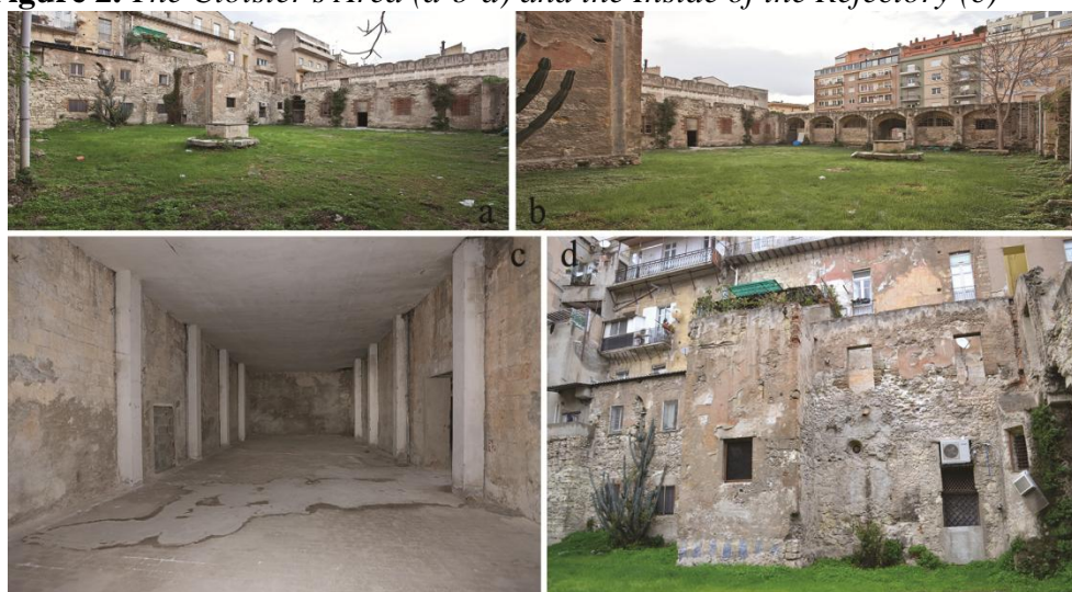
Figure 2. The Cloister's Area (a-b-d) and the Inside of the Refectory (c)
