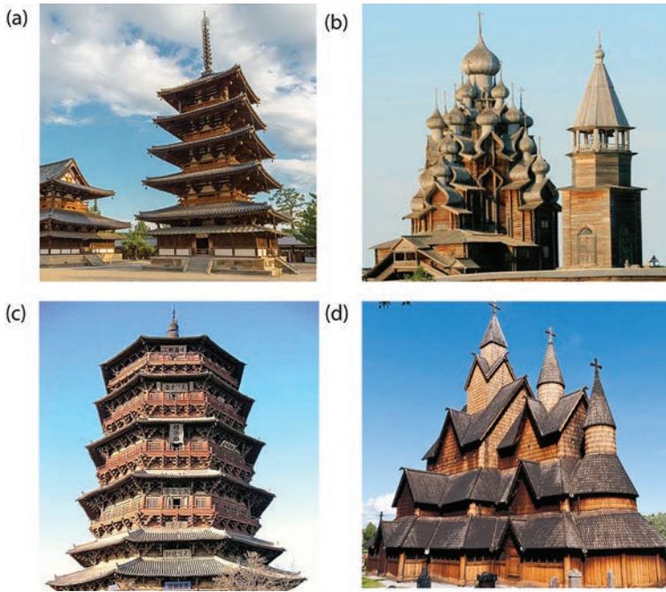
Figure 5. Ancient wood constructions: (a) Hōryū-ji Pagoda (Japan, 607 A.C.); (b) Kizhi Pogost Church (Russia, seventh century); (c) Fogong Temple Pagoda (China, 1056 AC); (d) Heddal stave church (Norvegy, thirteenth century).
