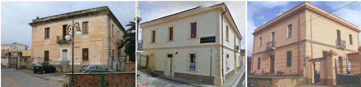
Figure 4. Carabinieri barracks in Sardinia (CA): the case of Ballao (abandoned), Villasalto (used for social activities) and Narcao (still military)
