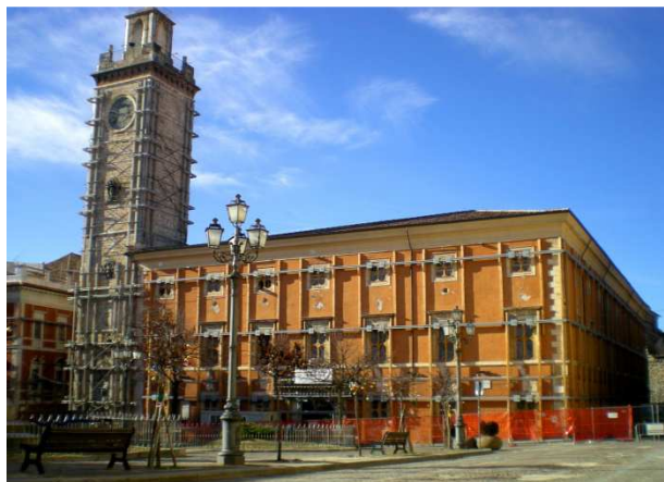
Figure 5. Post-earthquake temporary metallic bracing.
