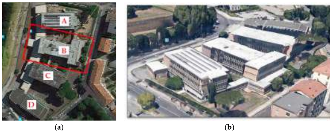
Figure 1. Plan (a) and aerial view (b) of the School Complex I.T.C. F. Carrara (Lucca–Italy).
