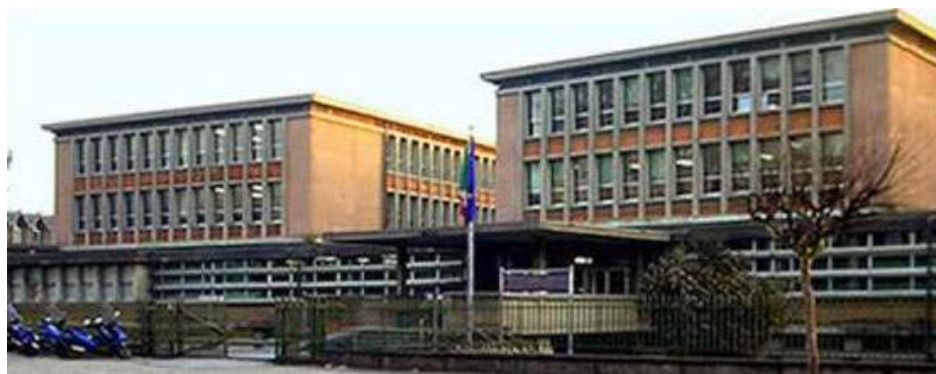
Figure 2. View of the B pavilion (right) and C pavilion (left).
