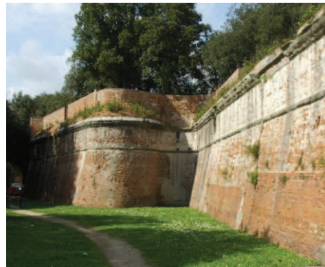
Fig. 2- Detail of the retired flank with orillon in the Fortezza Nuova of Pisa
