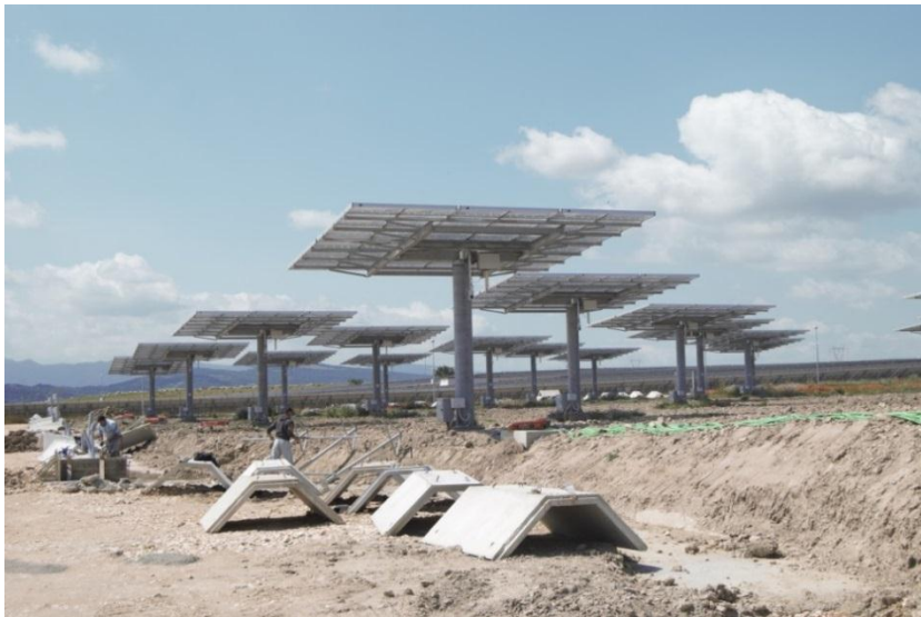
Figure 3.9. CPV field of the Ottana Solar Facility (under construction)
