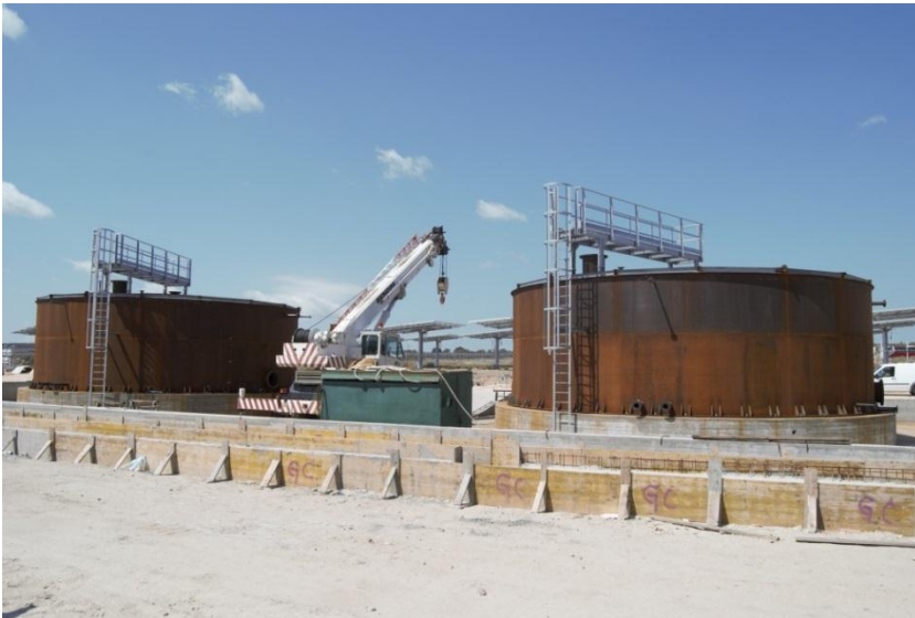
Figure 3.6. TES of the Ottana Solar Facility (under construction)
