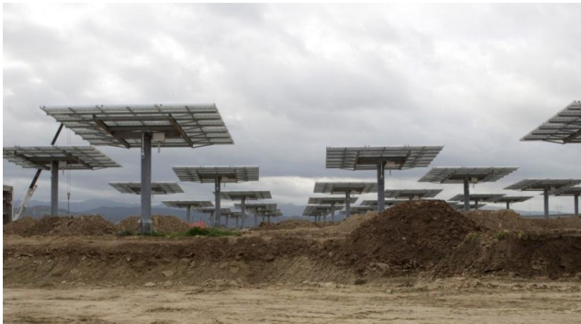
Figure 3.8. CPV field of the Ottana Solar Facility (under construction)
