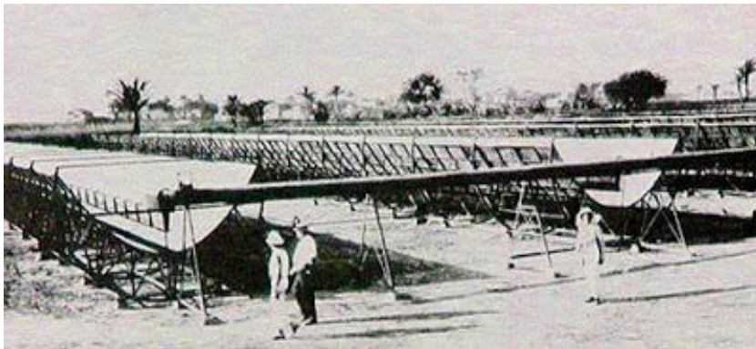
Figure 2.2. The very first CSP Plant in Egypt (source: The New York Times, published: 2 July 1916)
