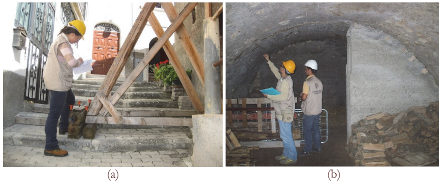
Figure 7: Students surveying structural features and damages of a building (a) and an hypogeal structure (b).
