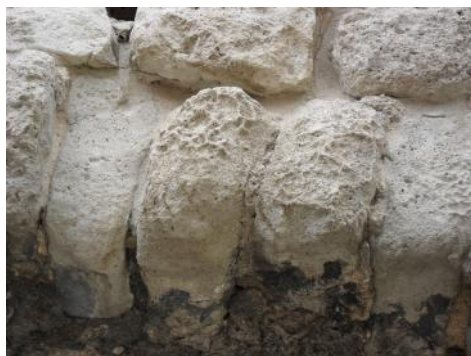
Fig. 4- Altered ashlars of inner vault of pentagonal tower (east facade) and the bedding mortars
