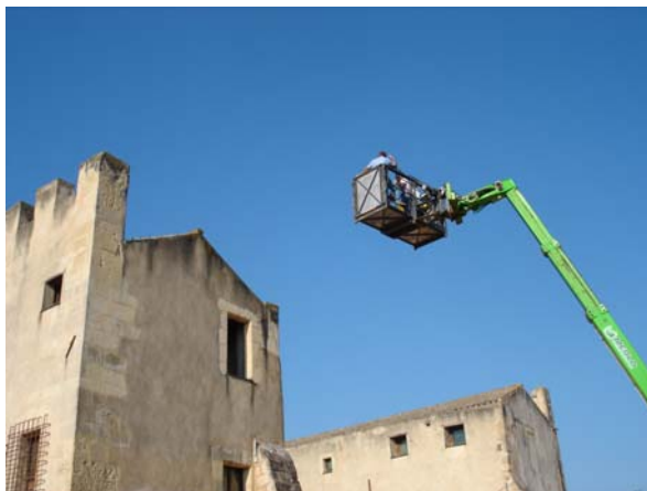
Fig. 8: Lifting platform to roof survey
