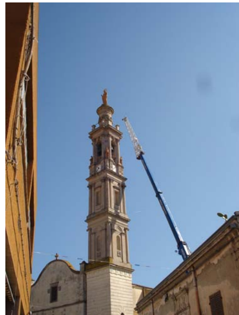
Fig. 13: Laser scanner survey of the Bell Tower
