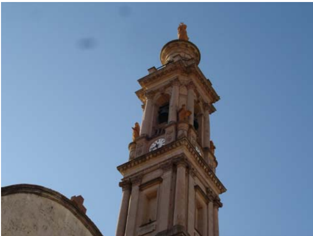
Fig. 2. Mores Tower Bell
